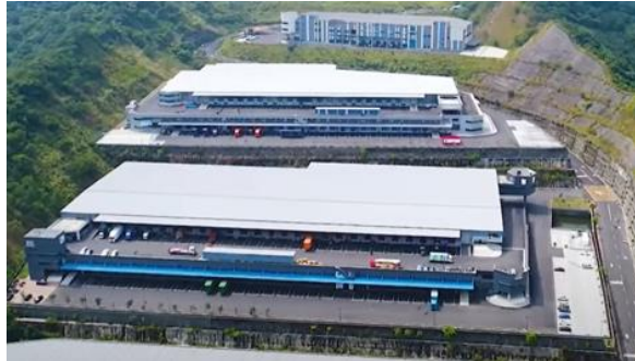
Facility in New Taipei City, Taiwan
